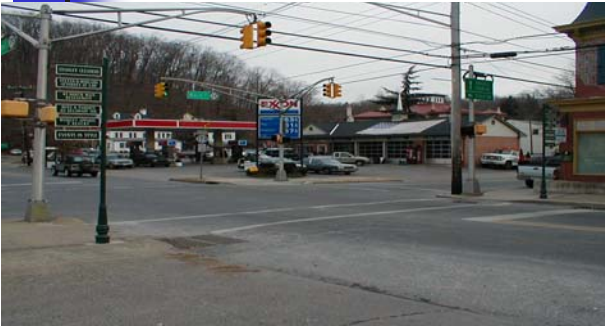
Route 29 Streetscape & Drainage Improvements
