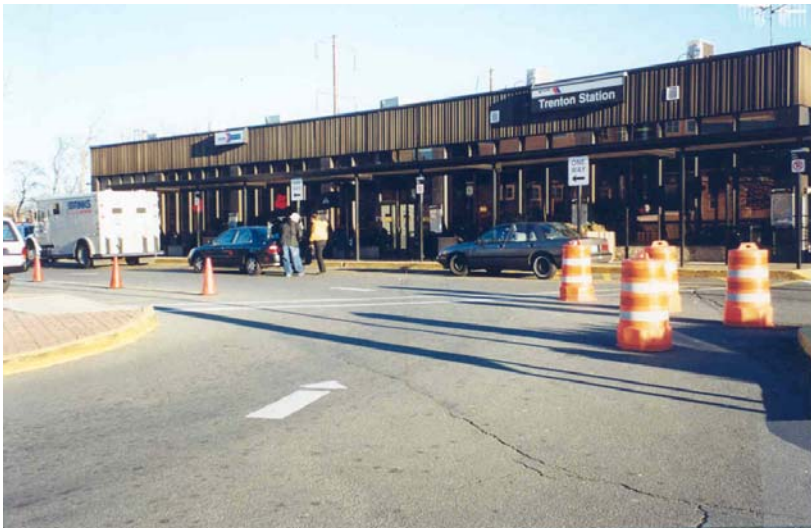
NJ Transit – Trenton Railroad Station Rehabilitation Project
