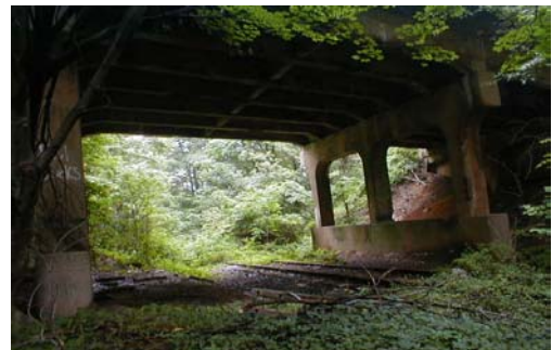
Route 33 Over Conrail Bridge Replacement
