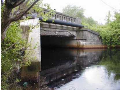
Route 70 Over Bispham's Mill Creek - Bridge Replacement
