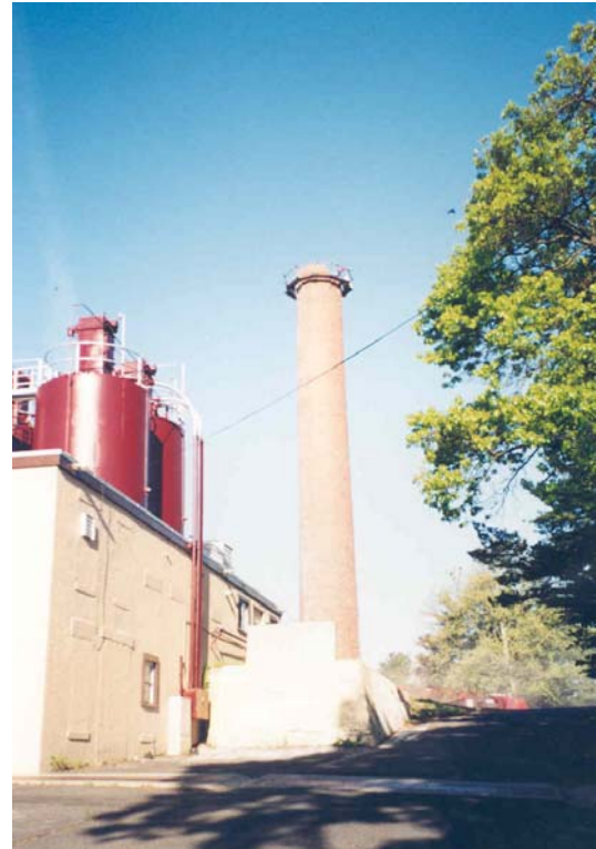
Demolition of Chimney near existing structure
