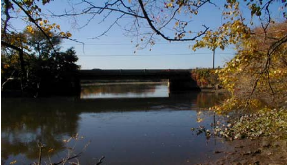
Bridge Scour Countermeasures South region
