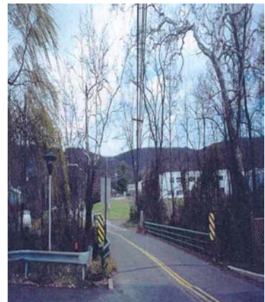
Newburgh Road Bridge Improvements
