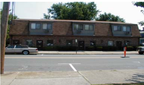
Mixed-Use Building, Lincoln Park, NJ
