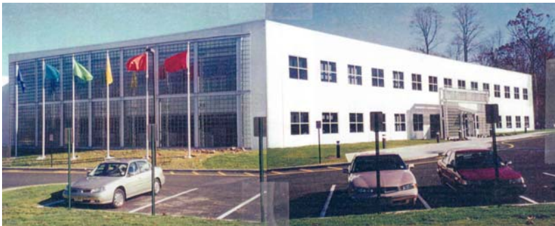
Konica Photo Imaging Facility, Mahwah, NJ
