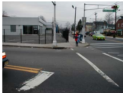
Route 82 Streetscape and Intersection Improvements
