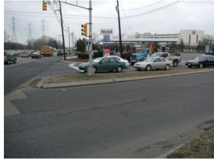
Route 1 Widening Project
