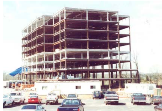
Somerset Corporate Center Bridgewater, NJ
