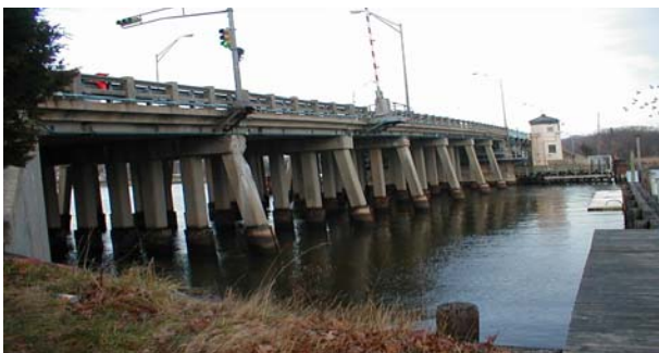
Route 70 Over Manasquan Bridge Replacement
