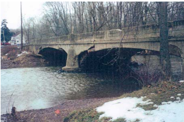
Amwell Road Bridge Improvements
