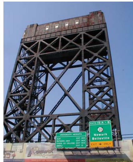
William A. Stickel Bridge Rehabilitation
