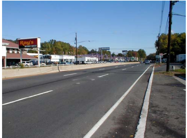
Route 22 Crab Brook Drainage Improvements
