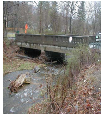
Sanatorium Road Over Spruce Run - Bridge Replacement
