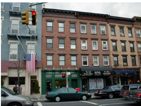
Commercial Building, Brooklyn, NY
