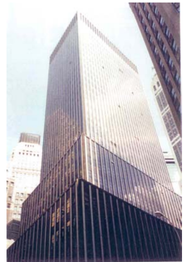
Office Building New York City, NY
