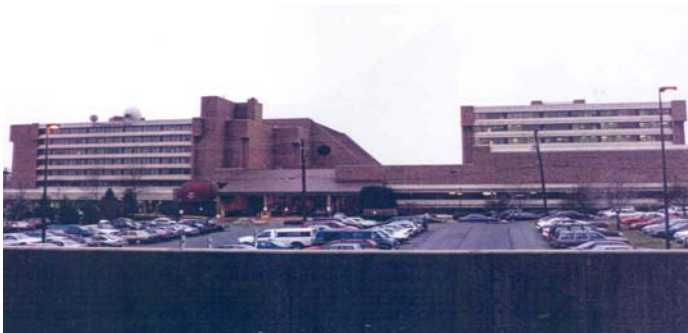
Twin Office Center, Rockville, MD
