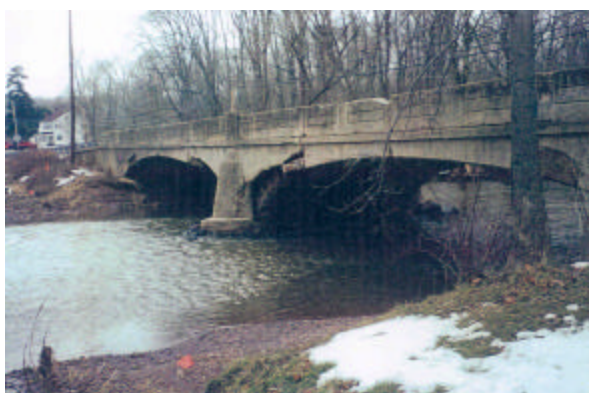
Amwell Road Bridge Improvements
