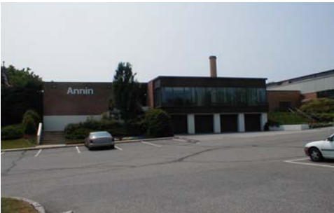
Industrial Property, Roseland, NJ
