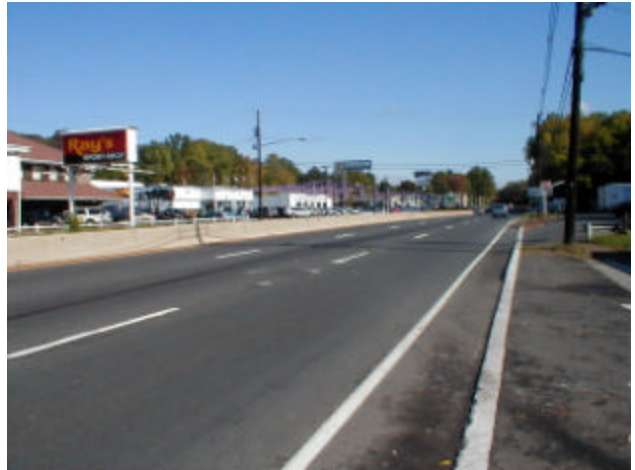
Route 22 Crab Brook Drainage Improvements
