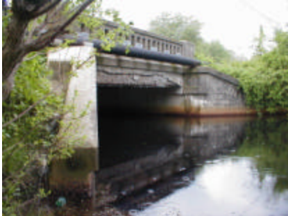
Route 70 Over Bispham's Mill Creek - Bridge Replacement
