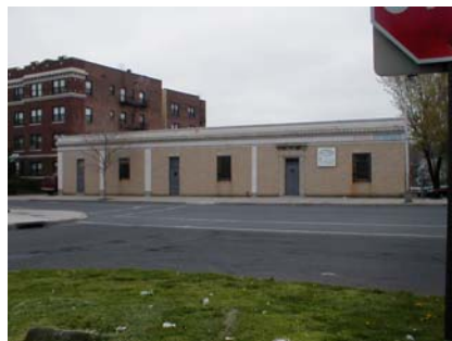
Family Development Center East Orange, NJ
