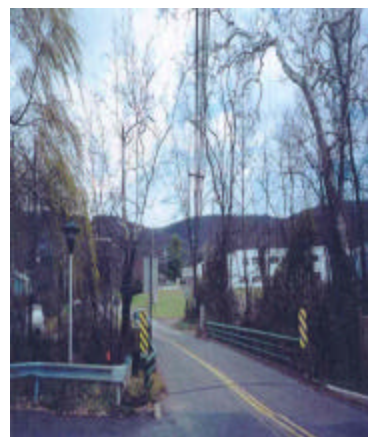
Newburgh Road Bridge Improvements
