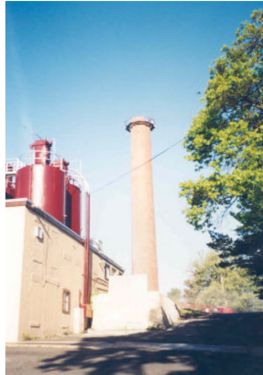
Demolition of Chimney near existing structure
