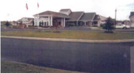
Oakmont Apartments, Webster, NY
