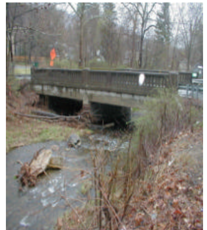
Sanatorium Road Over Spruce Run - Bridge Replacement
