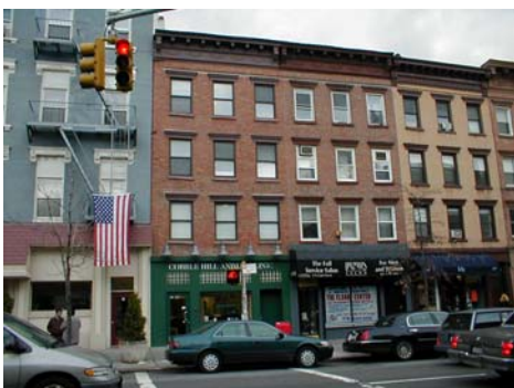
Commercial Building, Brooklyn, NY
